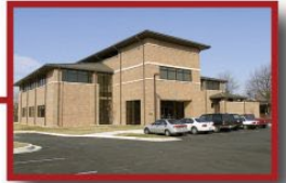
NNSS, Remote Sensing Laboratory - Andrews Joint Base Andrews, Maryland
